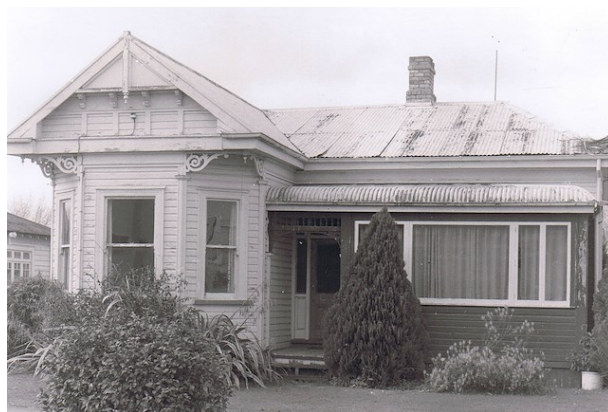
Dr Carolan's house much later in its life, just prior to demolition. MAH 0000.56.1
